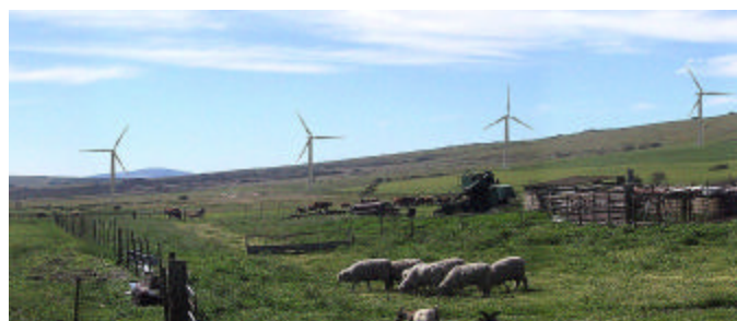
4 of the 10 wind turbines at Darling Wind Farm
