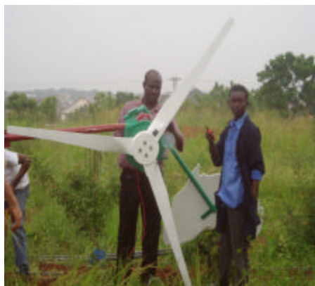
Ghanaian technicians prepare to erect a 2.4 metre diameter machine (Photo by Senyo Dake)
